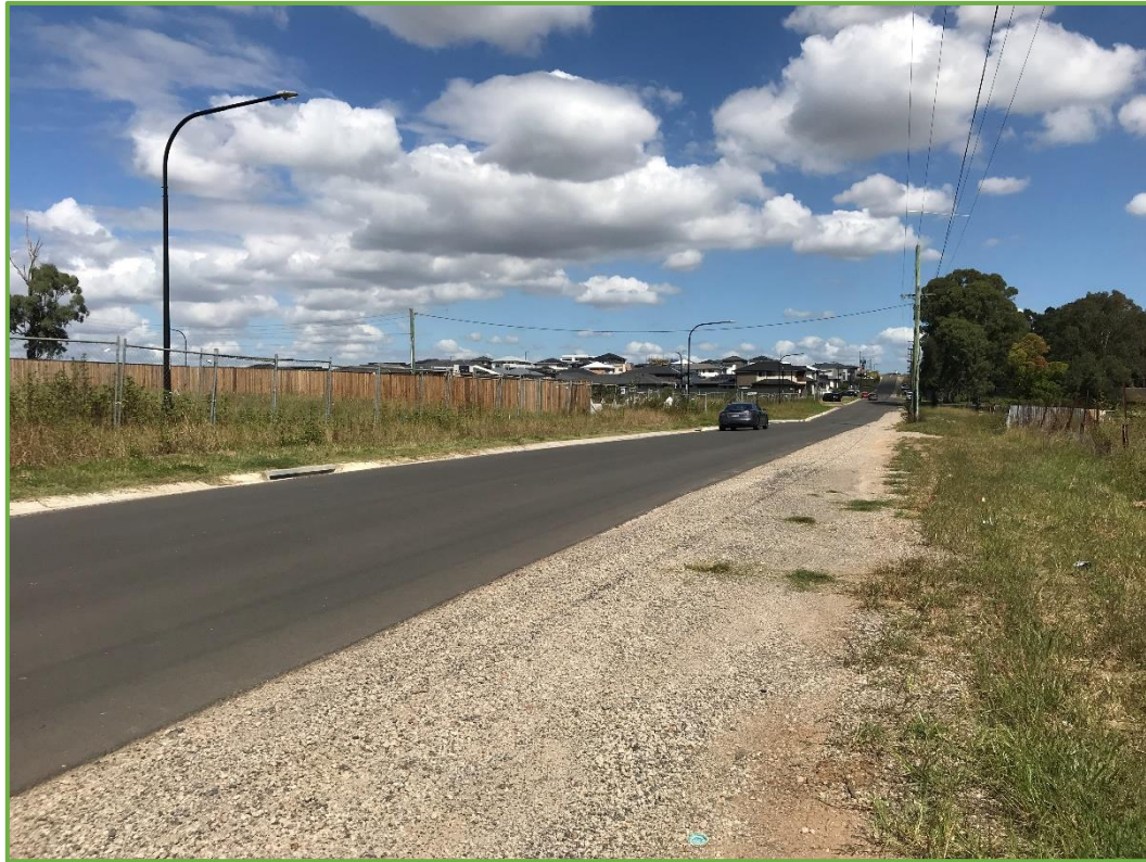
View looking west along Riverstone Road from the subject site's access driveway
